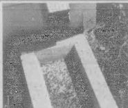
Problem: Washed-off shingle granules.
